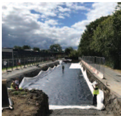
CRC flood defence work, Clontarf.
