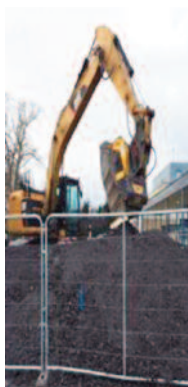
CRC flood defence work, Clontarf.
